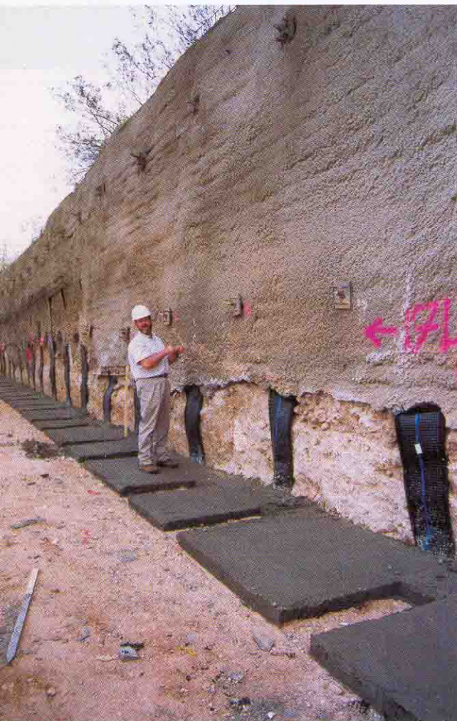
Bridge profile above with flash flood channel in foreground. Below photo shows formed concrete pads used to anchor walls.
