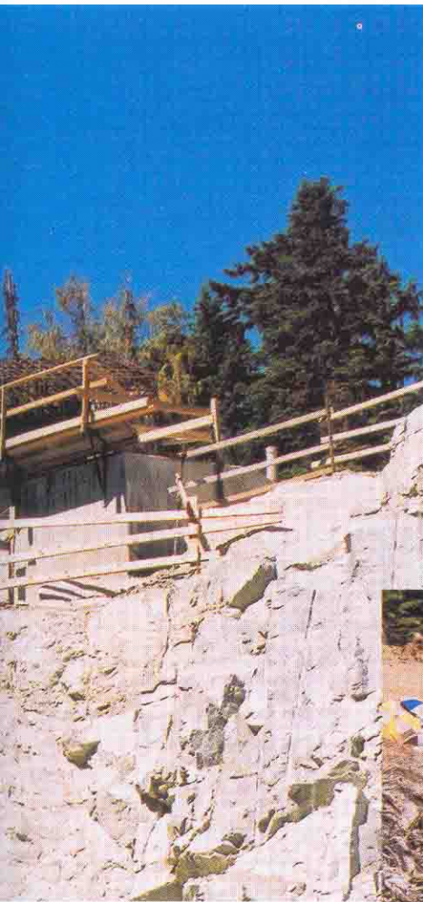
Photo on right shows construction of thrust block.
