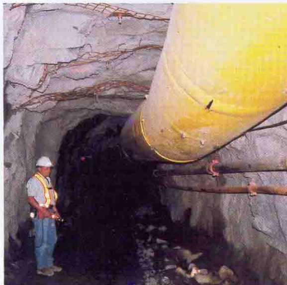
A close look at the 3 m x 2.75 m tunnel.
