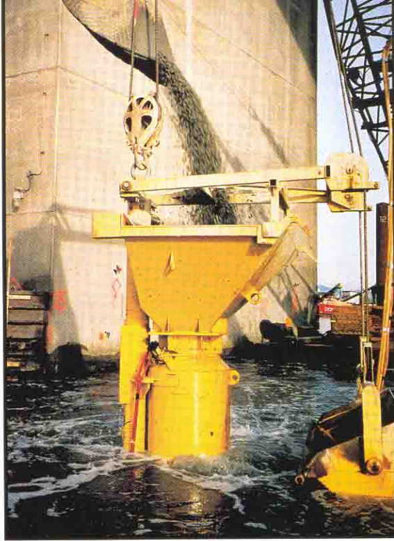
Stone being placed in new column near bridge pier.
