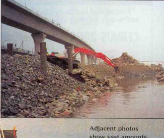
show vast amounts of dredged materials being stockpiled on barges while on shore, excavators place heavier materials close to Skytrain's elevated guideway.
