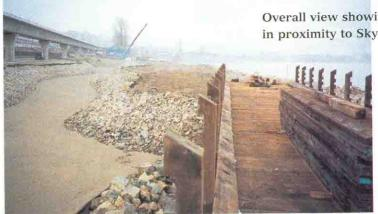
shoulder of the island up to the low water level. That part of the island was placed first to help contain the fines from the 152 mm minus that was used as general fill which makes up most of the rest of the island.
