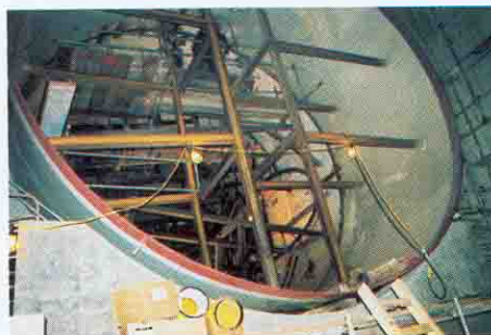
Fourth generation unit under construction.
