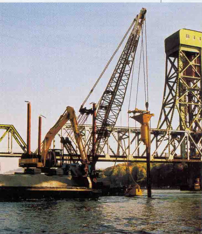
A crane and excavator work in tandem on pile installation.
