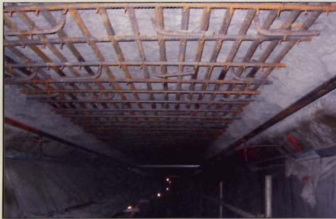
Above: Additional re-bar installed to the roof of the air duct
