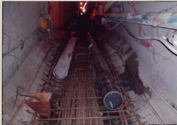
Above: Reinforcing steel added to the floor of the air duct
