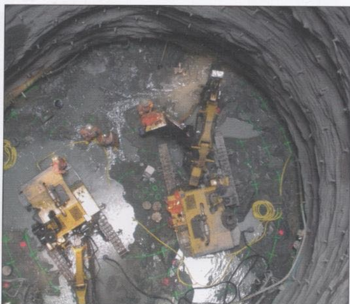
Mixed-face conditions complicated shaft sinking excavation
