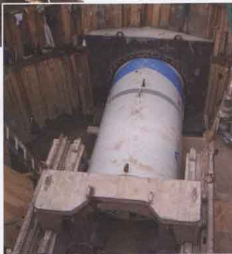
Right: Launch of the machine through the shaft's tunnel eye
