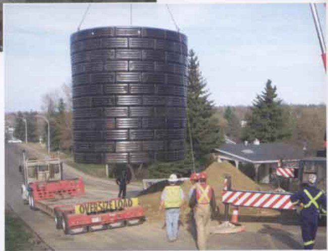
Below: A temporary bolted corrugated metal support liner used in the receiving shafts until removed for final construction of the manhole structure
