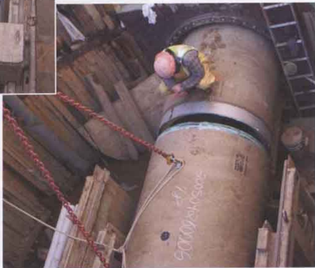
Jacking of the polymer concrete pipes selected for the contract
