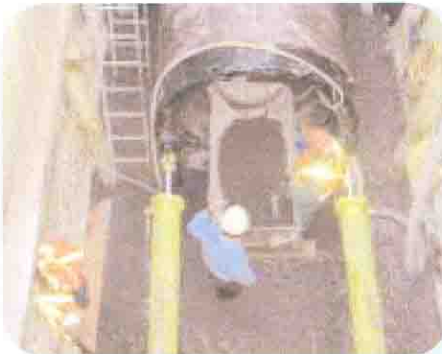
Pipe jacking under Highway No.1 for the 2L33 job.
