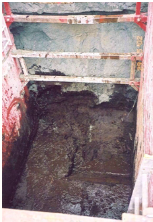
Soft Soils Excavation – very easy digging with obvious organic material and lots of groundwater
