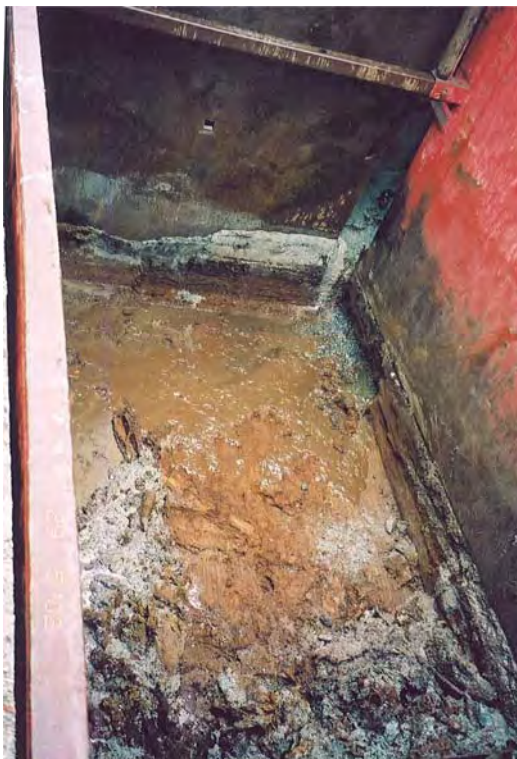
Soft Soils Excavation – very easy digging with obvious organic material and lots of groundwater
